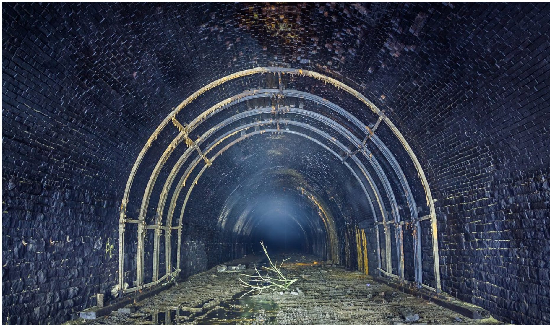
Section of arch ribbing with some laggings in situ. Spalled/wet/missing brickwork at crown.
