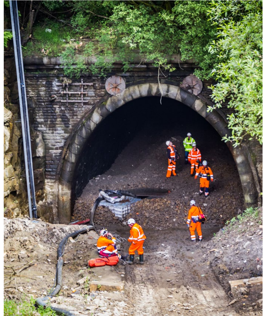
View of south portal after dewatering. Note pipework (left) for long-term pumping arrangements. Pumps are located in a sump in the tunnel entrance.
