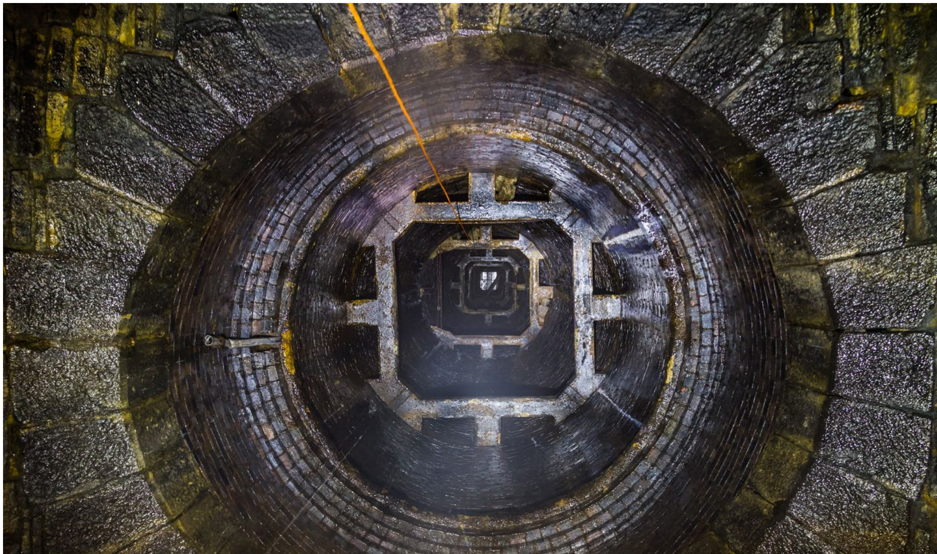
View up No.3 shaft showing brick relining and reinforced concrete frames, added for strengthening in 1934/5.
