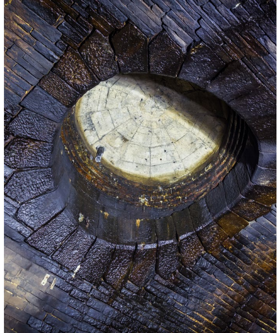
Concrete dome cap at base of No.1 shaft.
