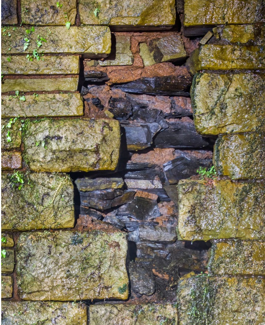
Missing stonework in D/S sidewall adjacent to the north portal.
