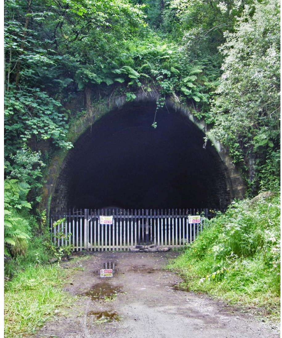
Contemporary photo of the north portal. Most of the parapet/copings are missing, as are the wing walls on both sides.
