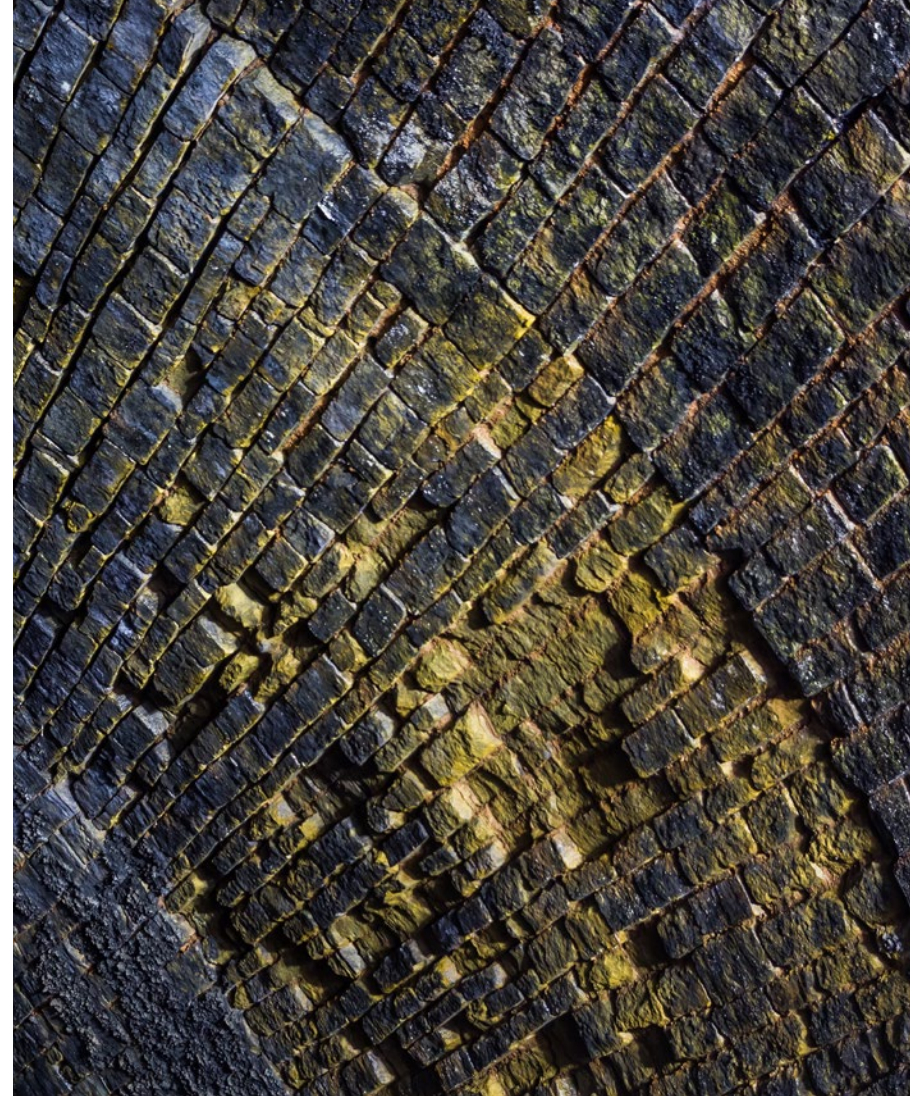
Spalled stonework and bulge at U/S haunch.
