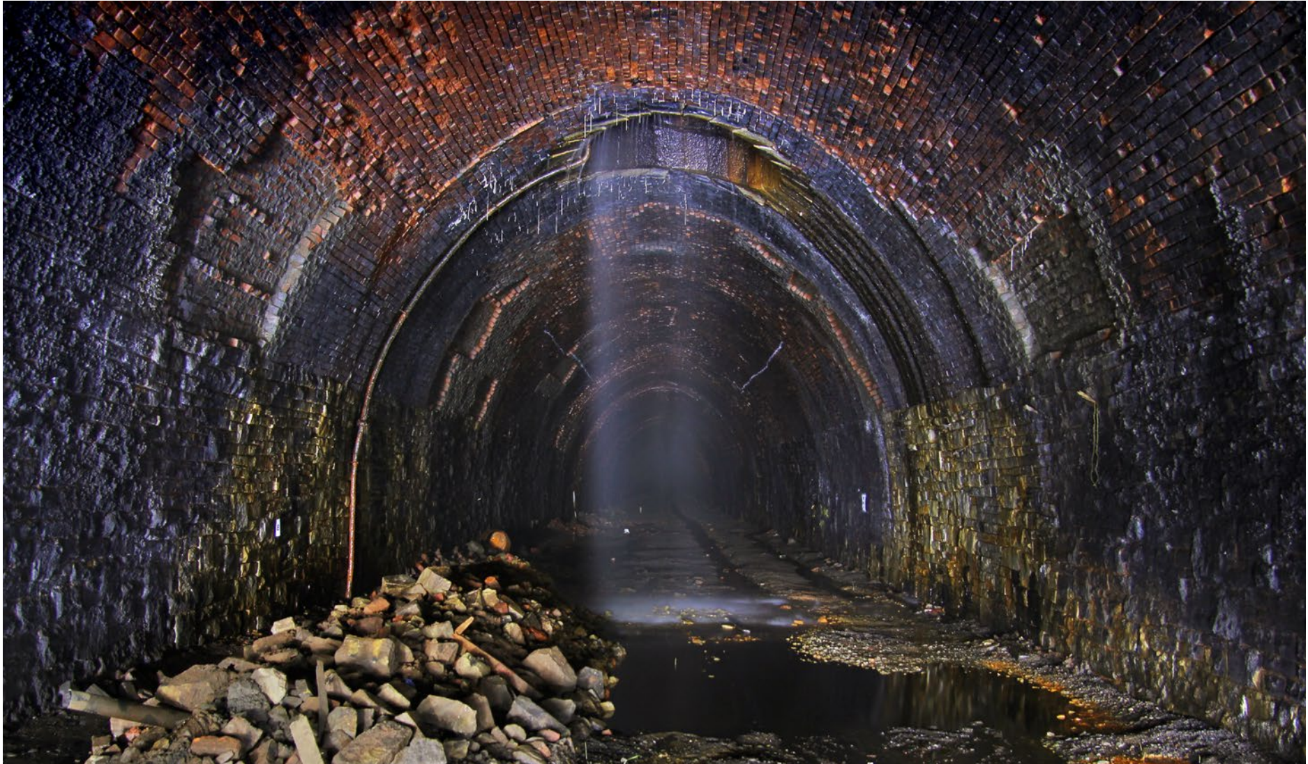
General view of No.8 shaft showing areas of missing brickwork. The arch at the other shafts is built in stone.
