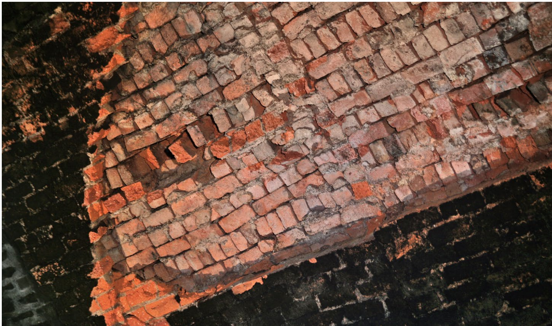
2007 view of missing brickwork at D/S haunch where collapse occurred in February 2013.
