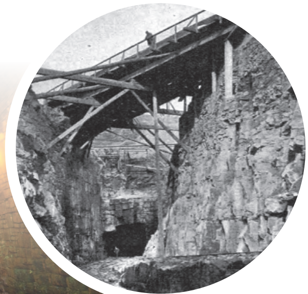
SOUTHERN ENTRANCE DURING CONSTRUCTION
